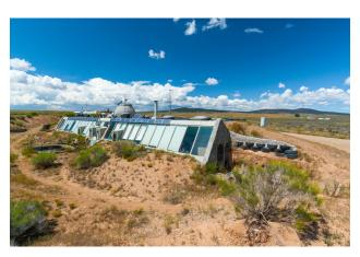
An <u>Earthship</u> is built out of the earth and a mix of recycled and reclaimed items, with energy-efficient and sustainable products for electricity, water, heat, cooling, and waste removal.
